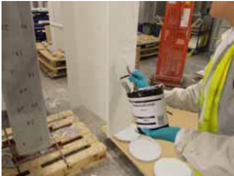
Interchar 2200 is easy to apply using a knife or trowel to repair damaged areas
